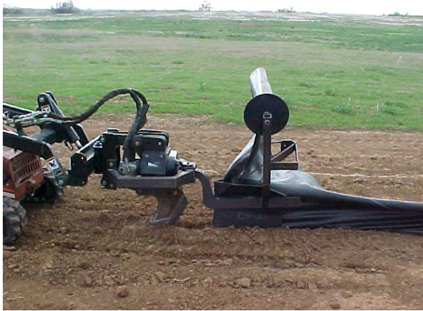
Figure 5. Tractor laying silt fence
