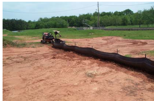
Figure 9 Silt fence attached to posts
