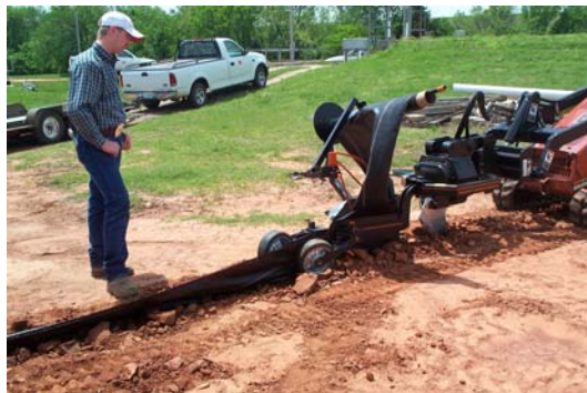
Figure 8 Installing silt fence with vibratory plow
