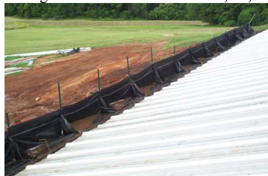
Figure 6 Water and sediment impounded between the flow barriers
