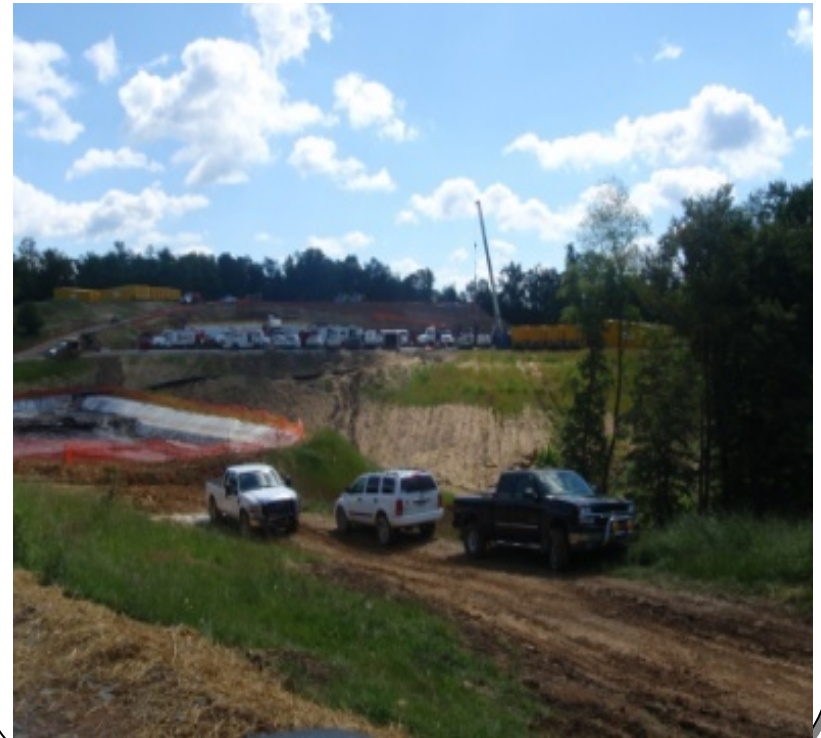
Bring Hydraulic Fracturing Equipment On location (Fayetteville Shale):
