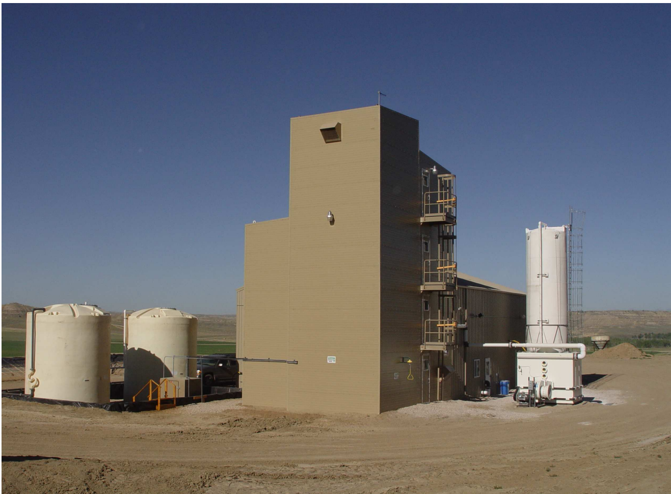
Single Treatment Unit 25,000 BPD Capacity
