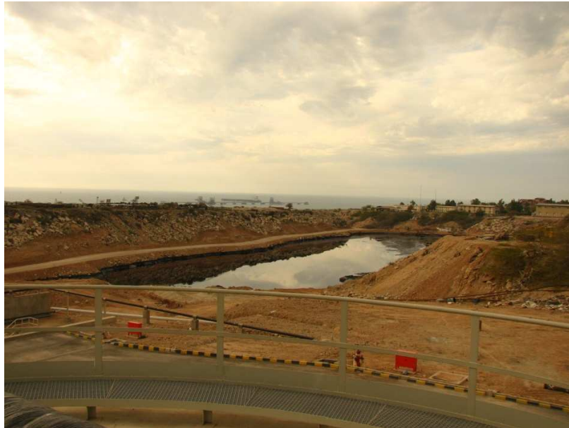
Figure 1. Retention pond for oil-water separation, Kharg Island, Persian Gulf, South of Iran
